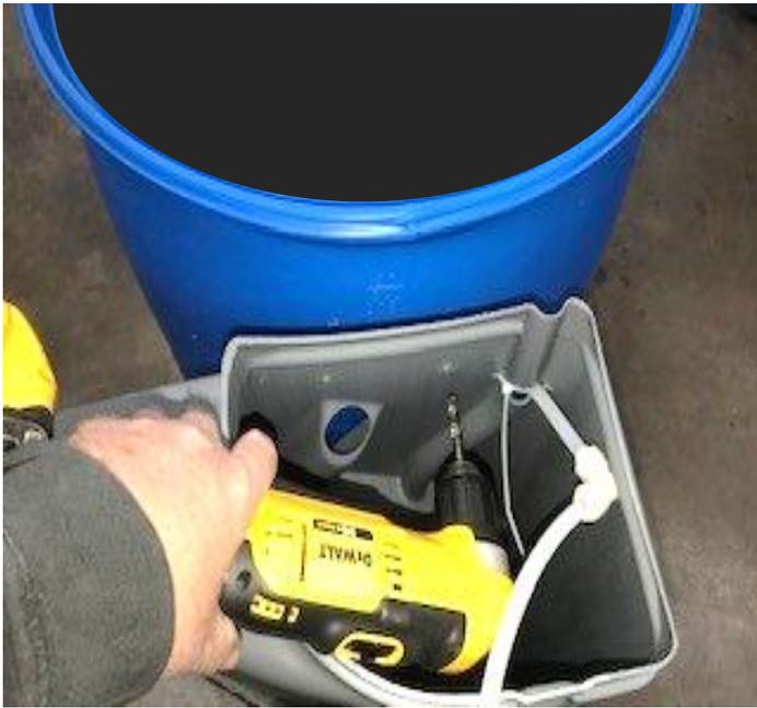
4) Drill the 30mm hole with the 30mm hole saw through the barrel.
